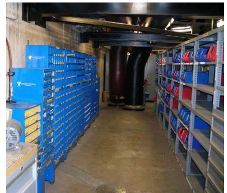
Spare Parts Storage
