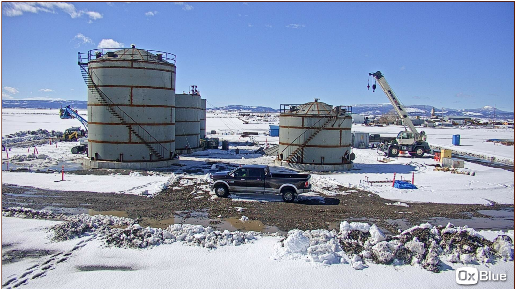
View of field fabricated tank construction, 28Feb2019, 1:30pm, facing W
