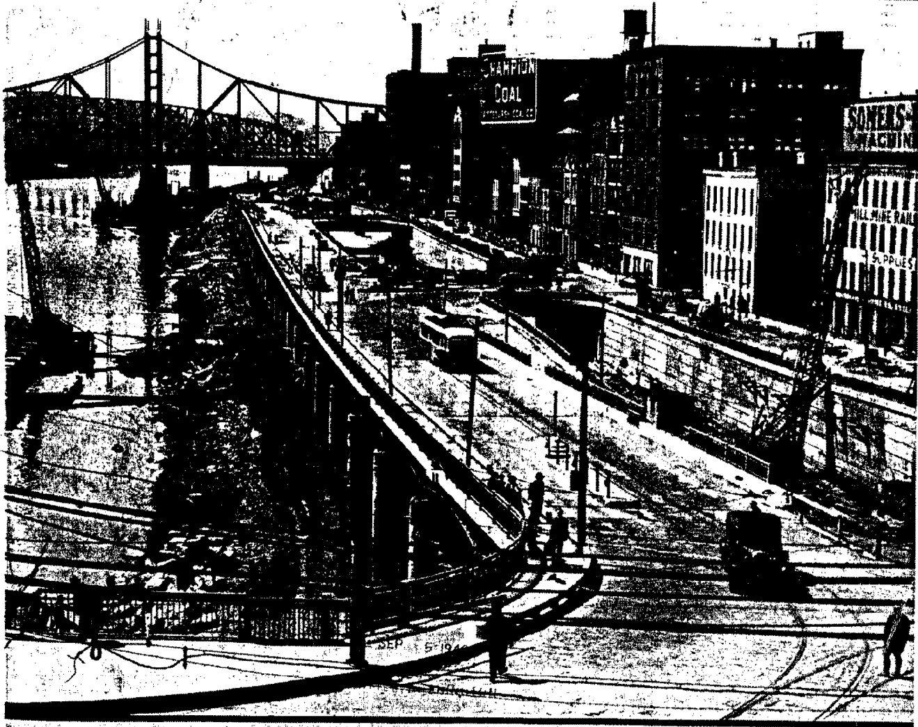
FIRST OF A SERIES OF IMPROVEMENTS PLANNED TO RELIEVE TRAFFIC CONGESTION IN PITTSBURGH'S GOLDEN TRIANGLE New Water Street Project, to Be Completed This Fall, Will Replace a 35-Ft Pavement with a Modern Highway of Ten Lanes
