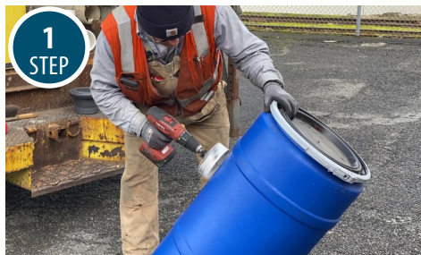
1 STEP Drill a 5-inch hole in barrel in the side of the barrel for a drain. Approximately 18 inches from the top of the barrel.
