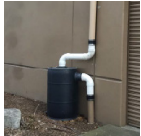
Oyster barrel in place at Terminal 102
