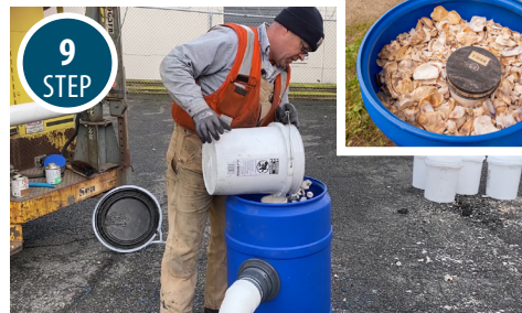
9 STEP Fill with 25-30 gallons of cleaned crushed oyster shells, about 2-3 inches below the interior overflow pipe.
