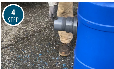
4 STEP Install 4-inch schedule 80 PVC threaded nipple on to bulkhead fitting.
