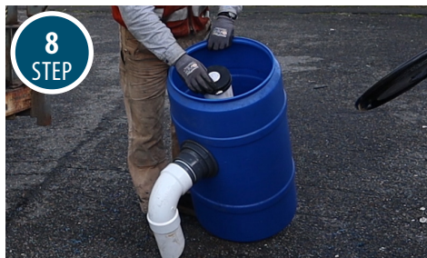
8 STEP Optional: used only if the overflow part of the tee inside drum is not going to be utilized.
