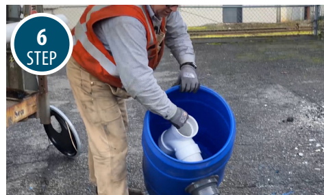
6 STEP Install interior piping to the bulkhead fitting.
