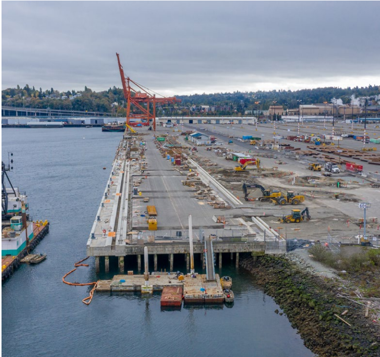
New north Berth at Terminal 5.
