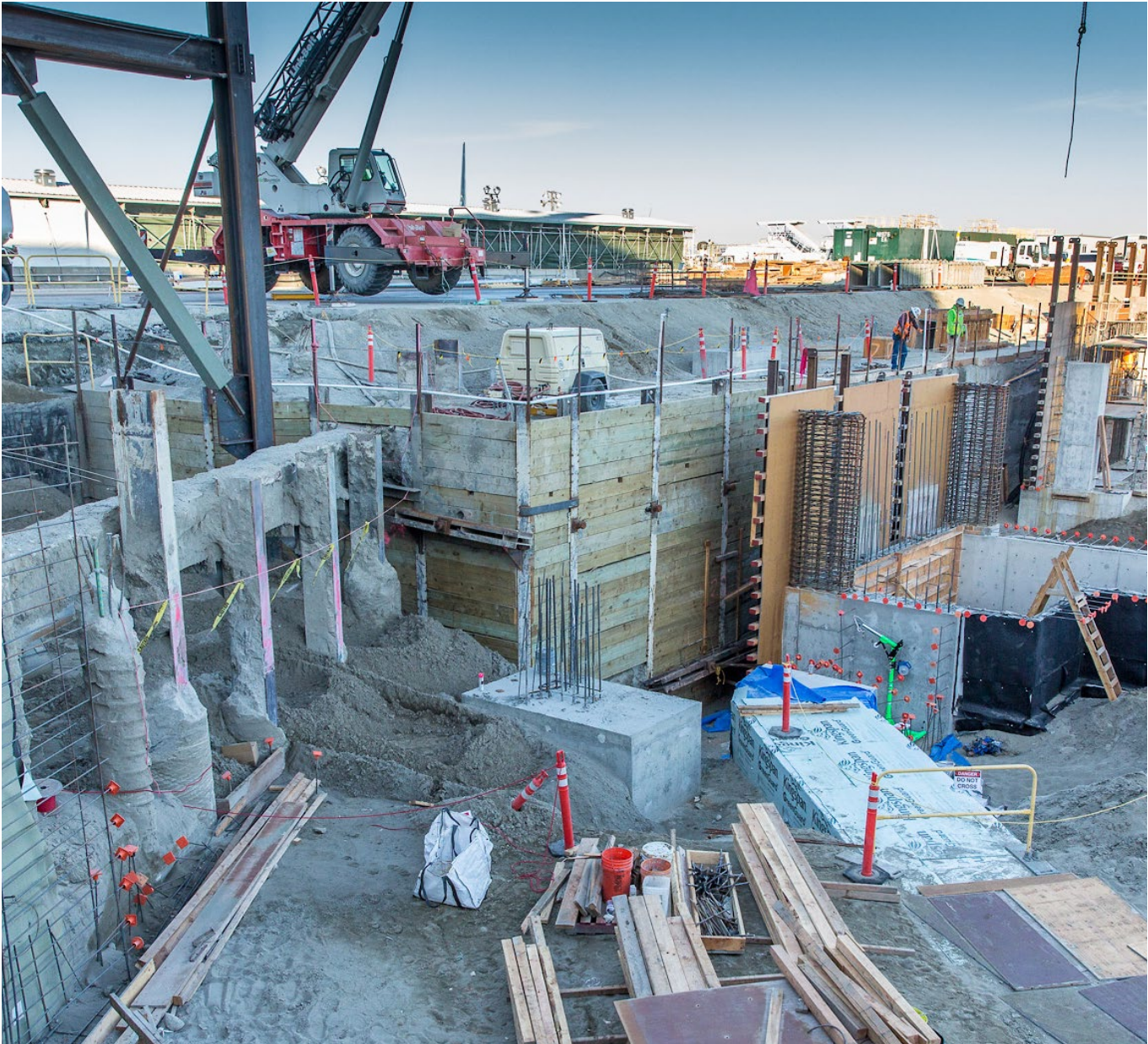
Excavation during the North Satellite Modernization Project.
