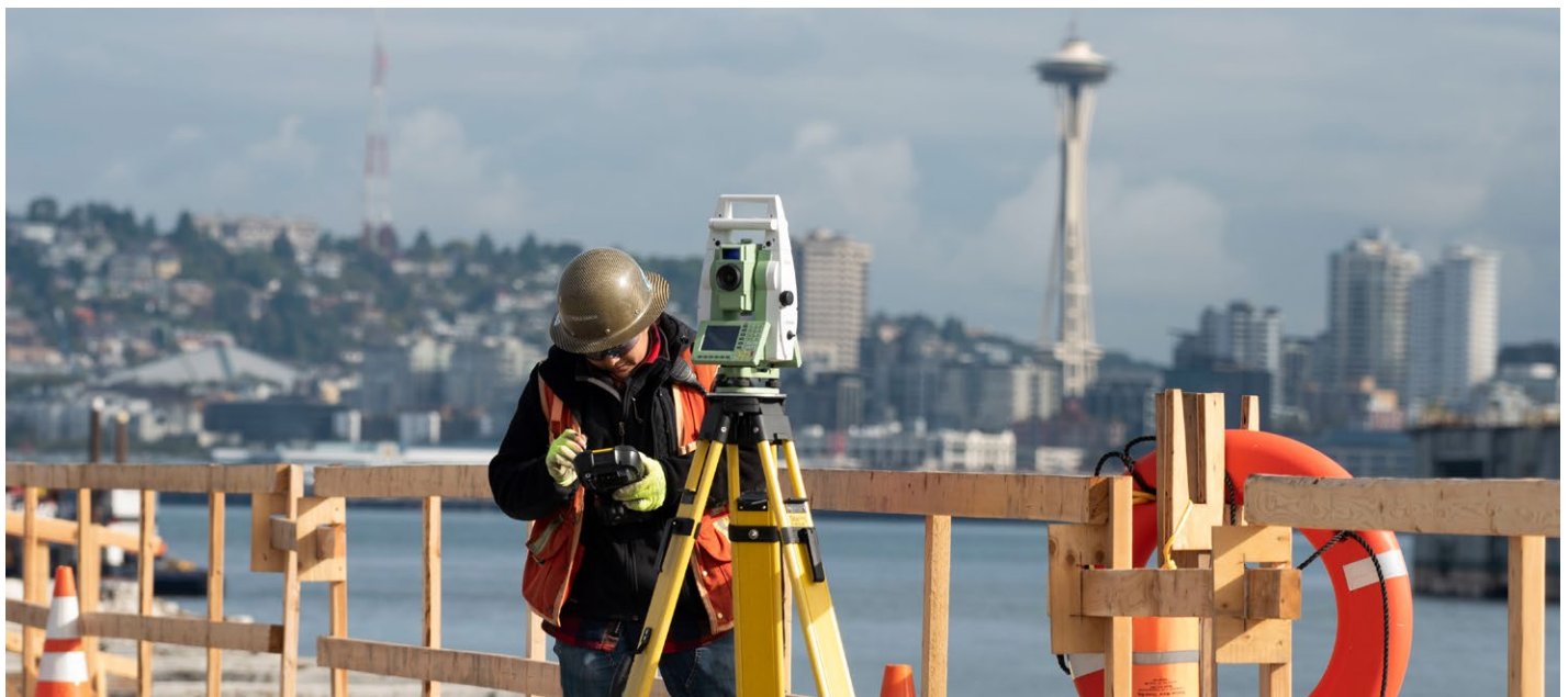
Surveyors working on the Terminal 5 Modernization Project.
