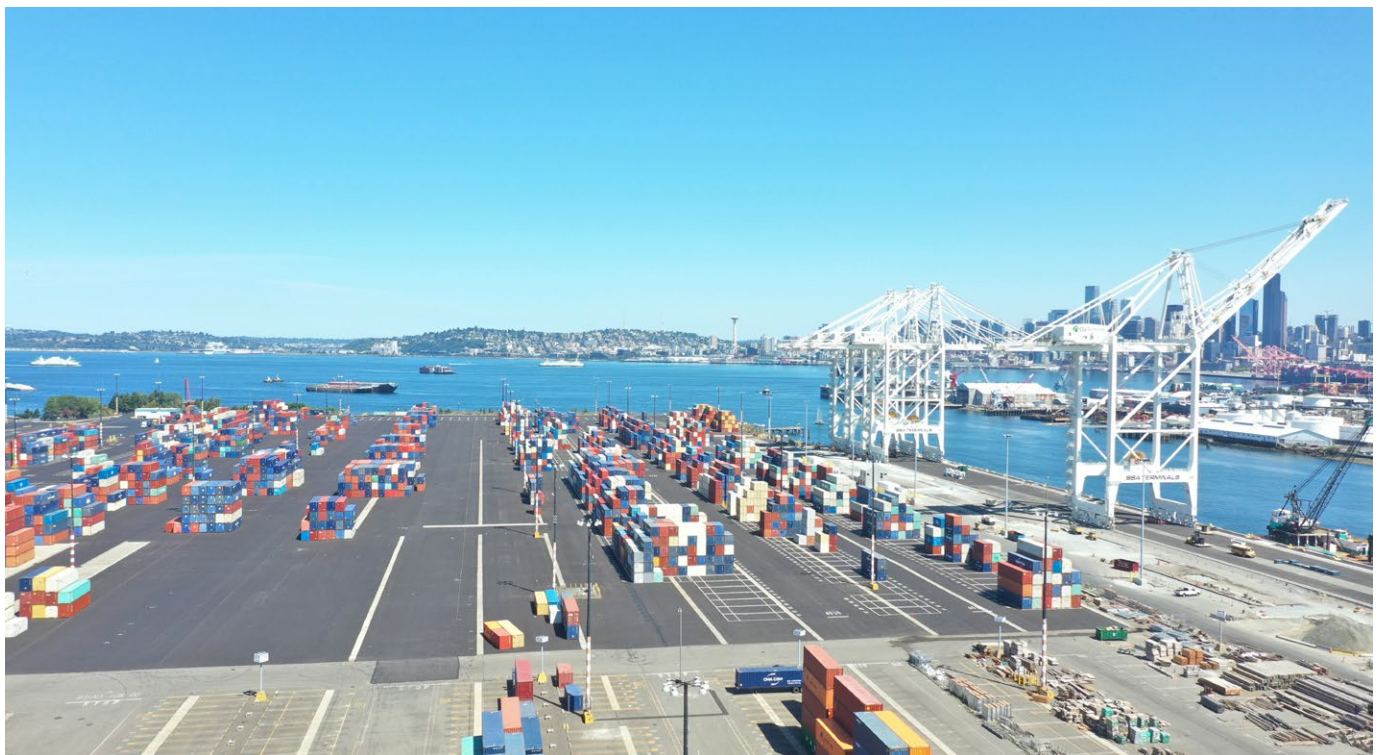
SSA Cranes at Terminal 5, part of the Terminal 5 Modernization Project.
