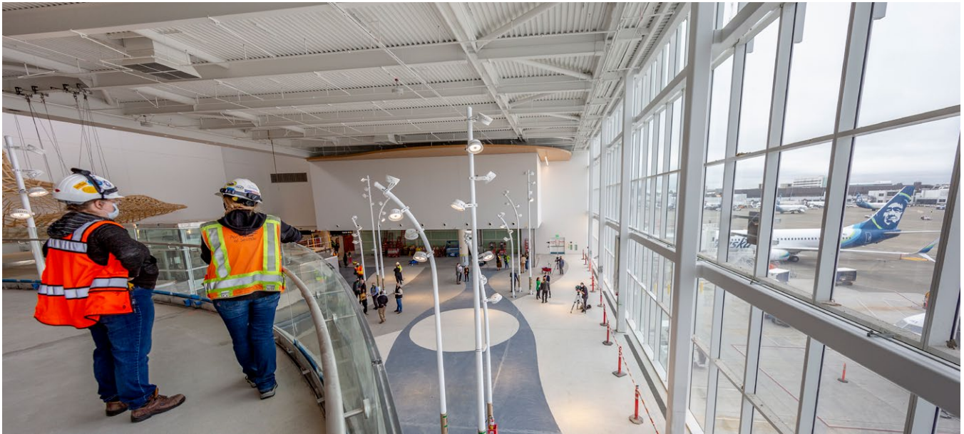
North Satellite Modernization Project almost complete.
