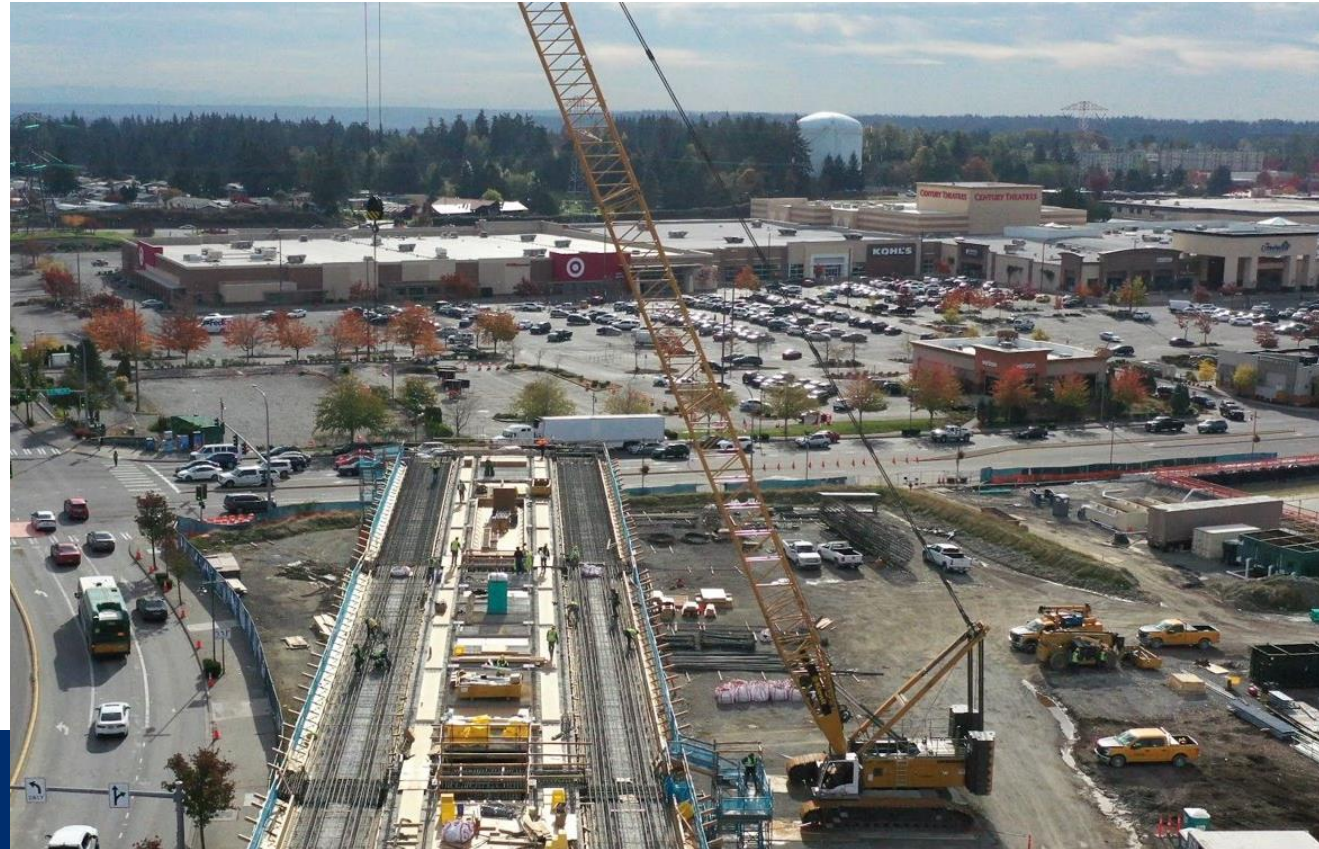
Right: Aerial photo of station platform construction, looking south
