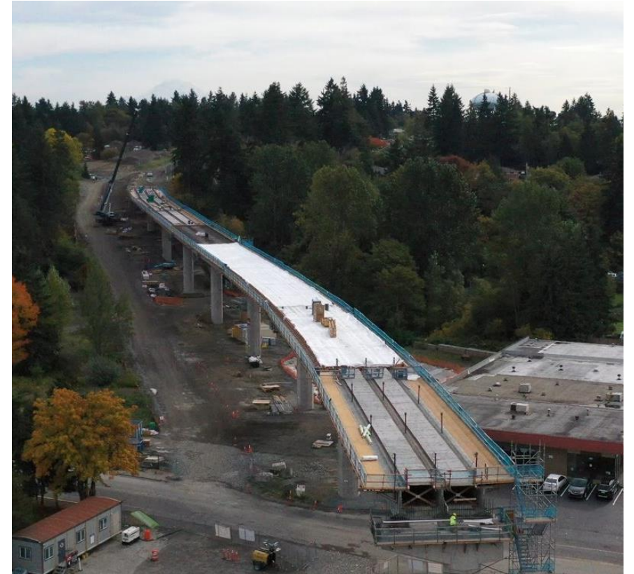
Above: Aerial photo of guideway construction in SeaTac
