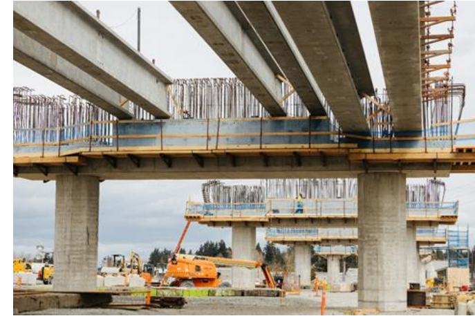
Federal Way Link Extension
