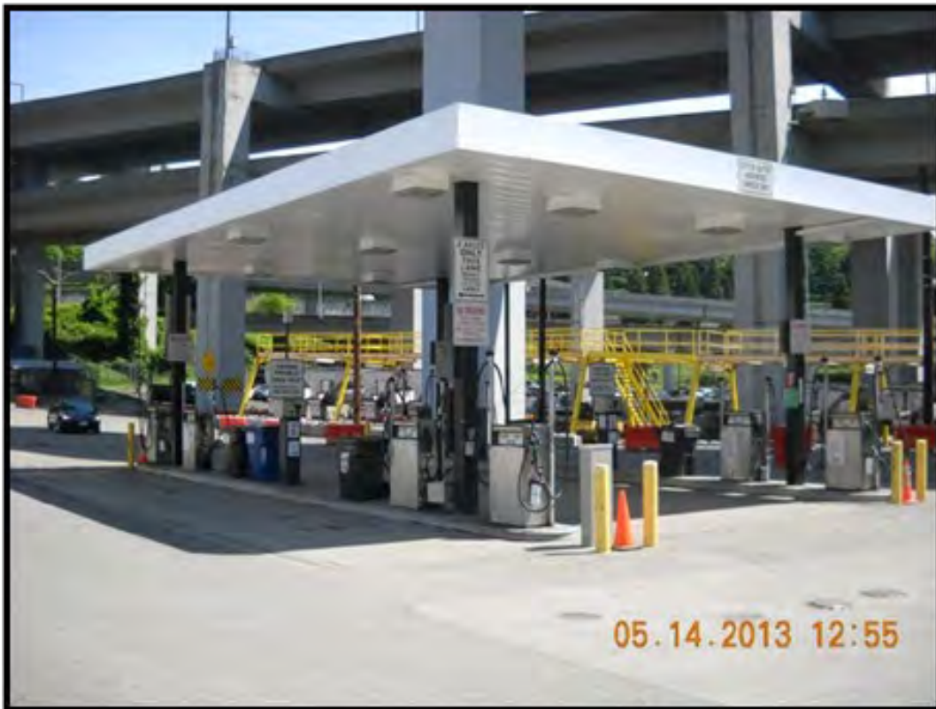
Figure 4. Roof at Fueling Island to Prevent Stormwater Run-On.
