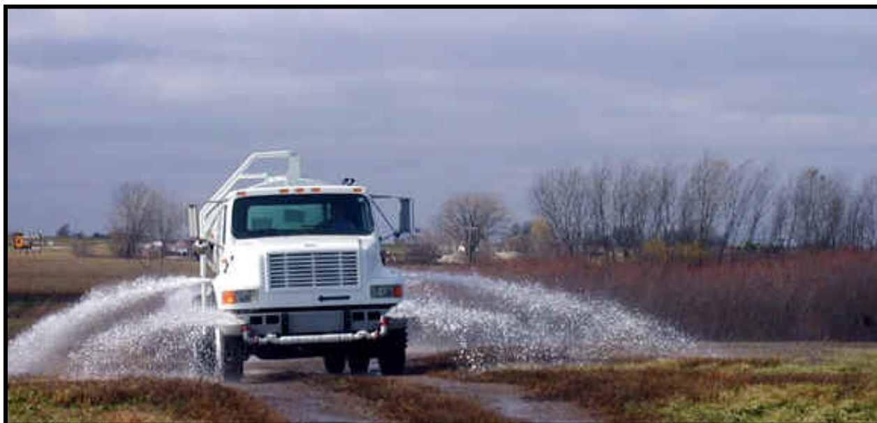
Figure 11. Using a Water Truck for Dust Control.
