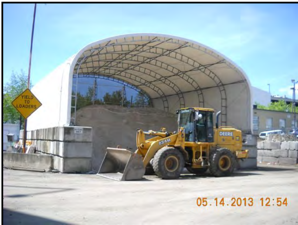
Figure 12. Covered Storage Area for Erodible Material (gravel).
