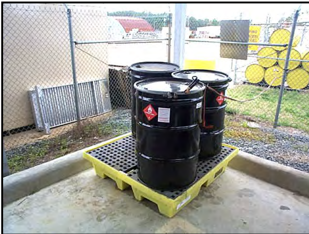
Figure 14. Containers Surrounded by a Berm in an Enclosed Area.
