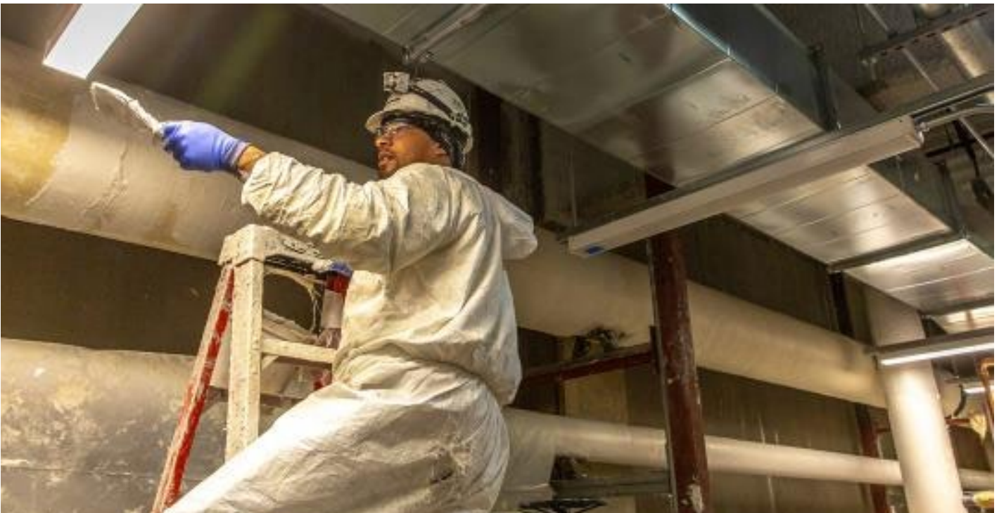
Work on the North Satellite Modernization Project.
