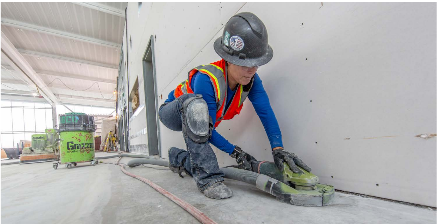
International Arrivals Facility Construction.
