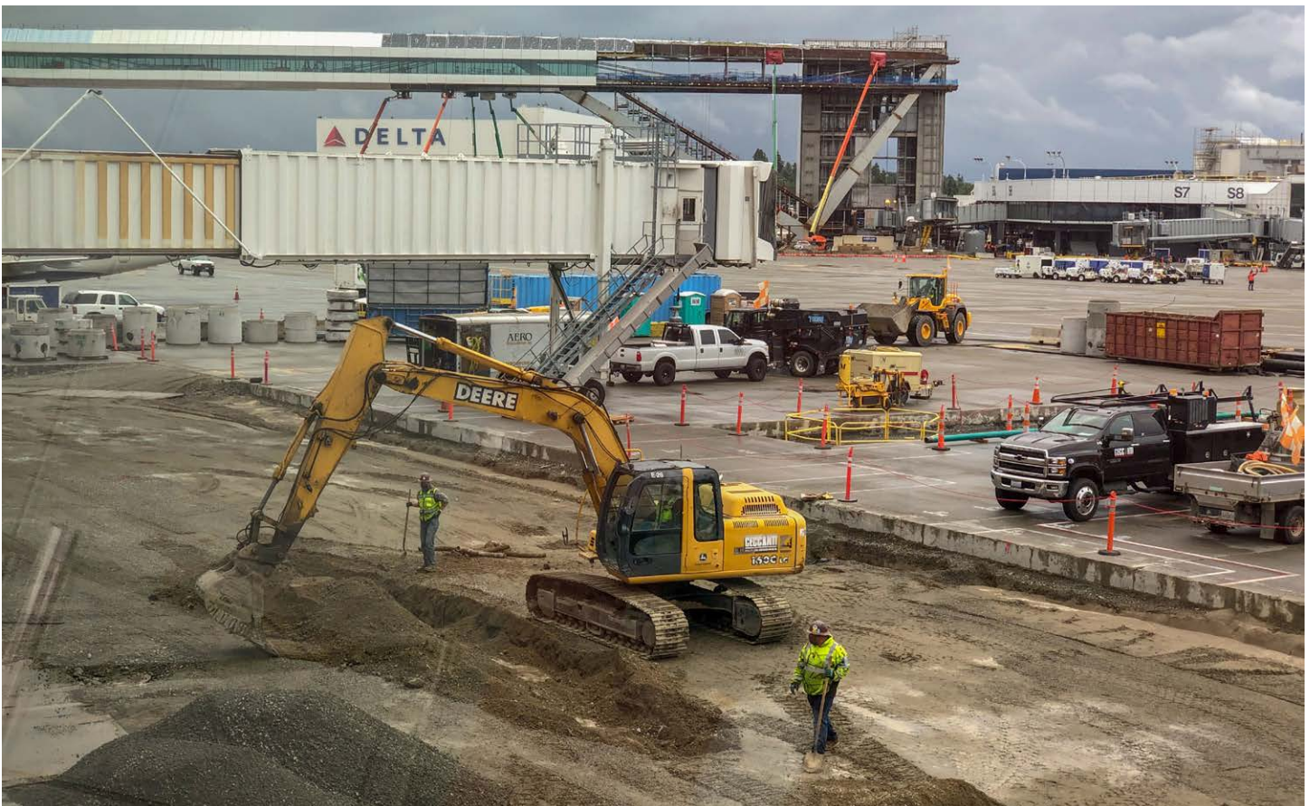
A Concourse Pod construction.
