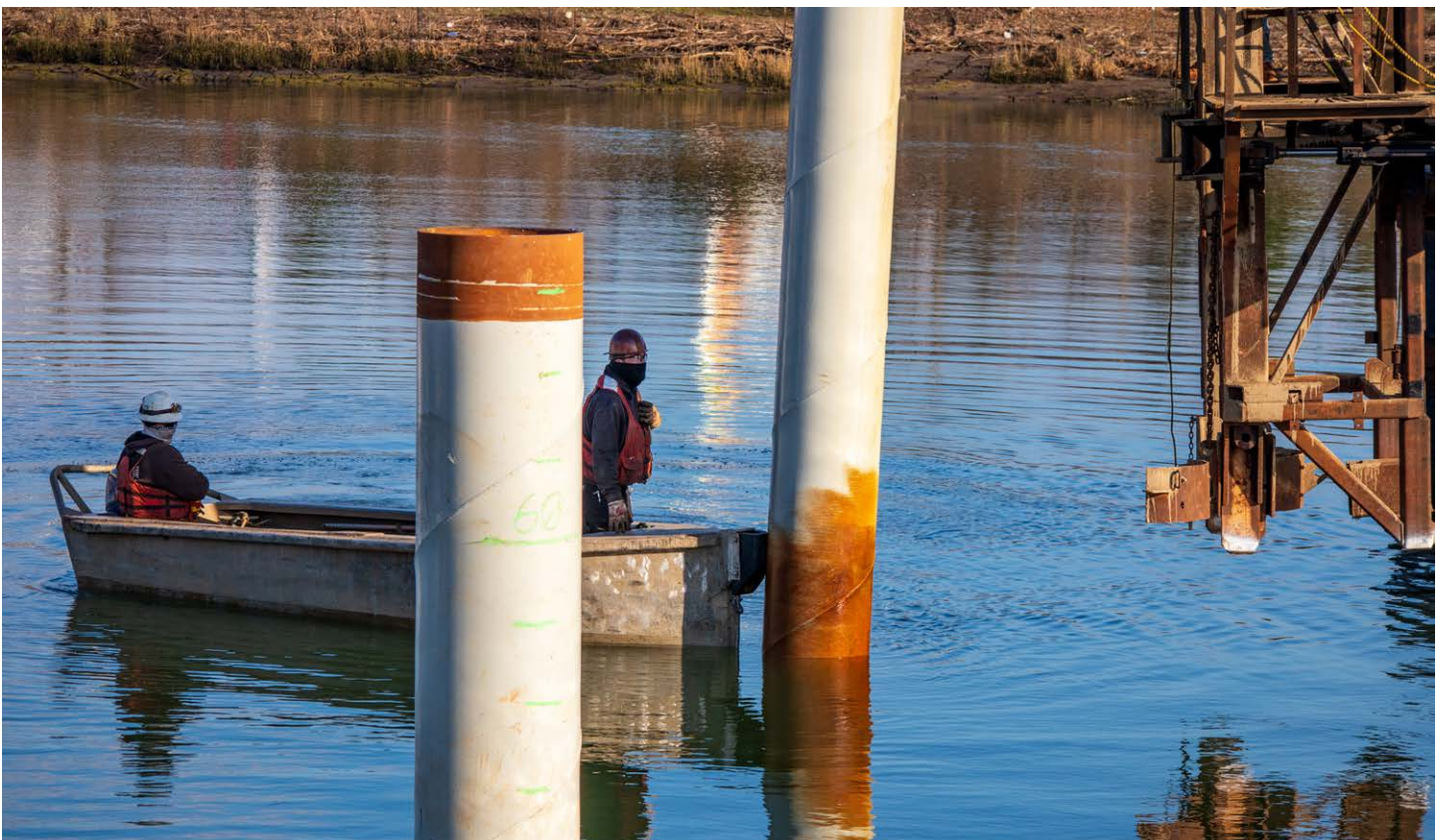
Pile driving on the Duwamish River People's Park.
