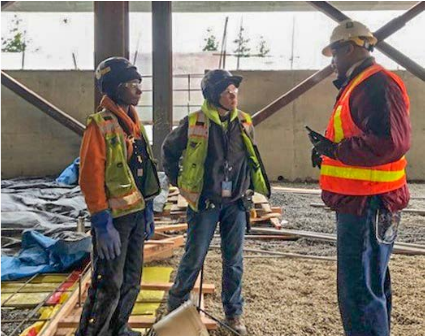
Interns on the North Satellite Modernization Project.
