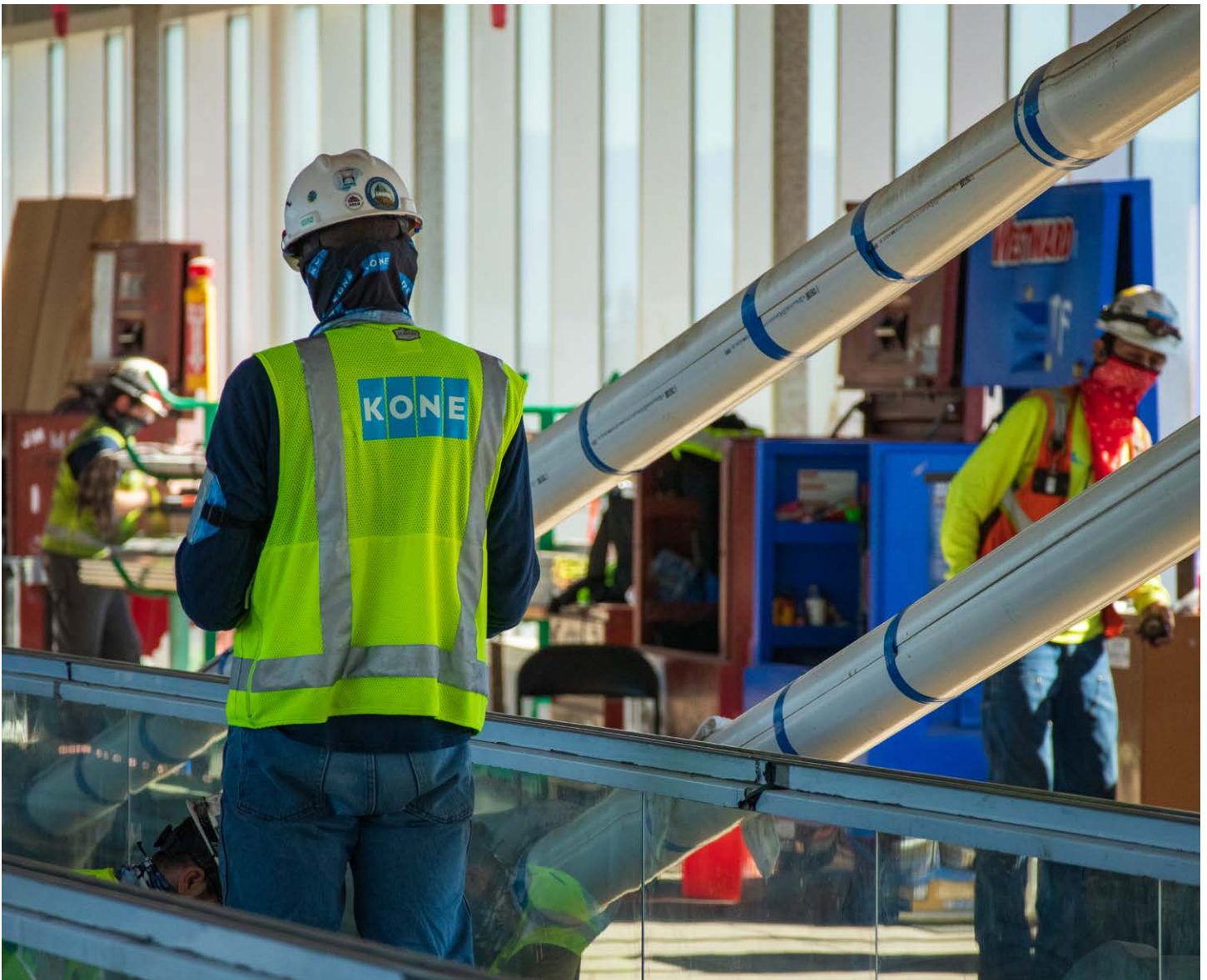
Construction on the Passenger Walkway on the International Arrivals Facility.
