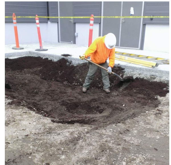
Example soil preparation: subgrade preparation
