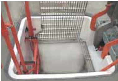
D-38 Vault Access Cover (965mm by 965mm opening)
